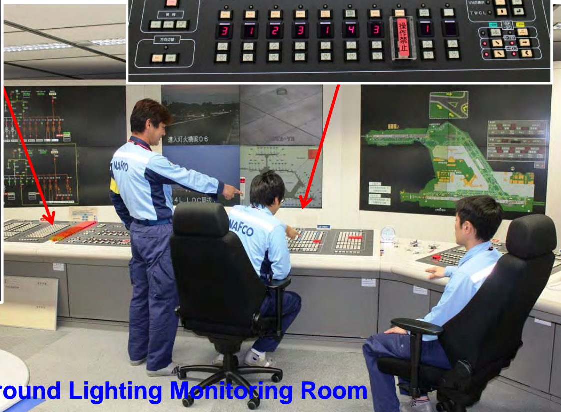
Aeronautical Ground Lighting Control Console
