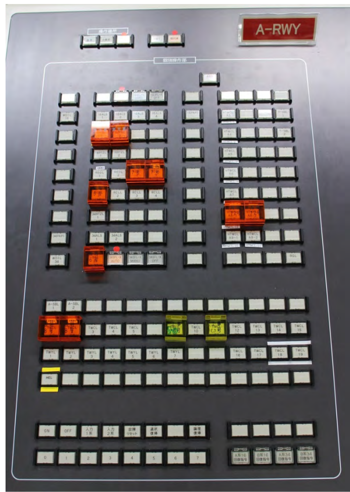
Aeronautical Ground Lighting Control Console
